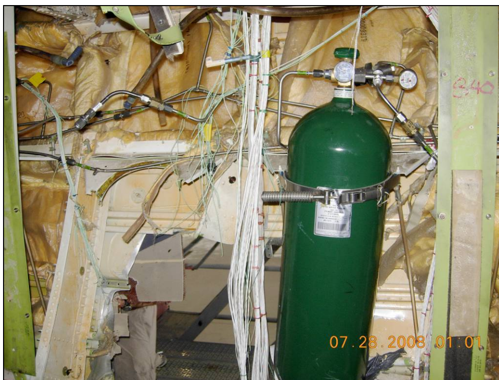
Figure 8: Number-5 oxygen cylinder adjacent to fractured fittings and lines from the number-4 cylinder
